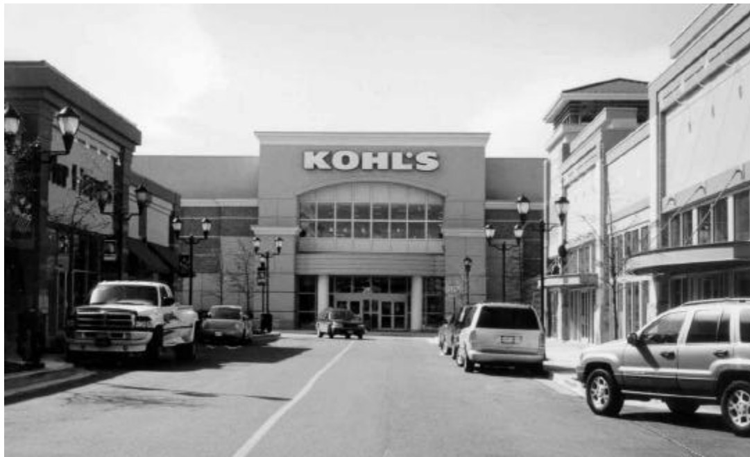
Kohl's is one of several big-box retailers located in the Washingtonian Center. Big-boxes are designed within a "main-street" environment.
